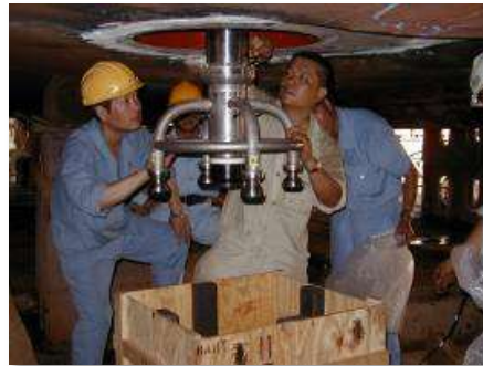
Deployable array on a hoisting system.
